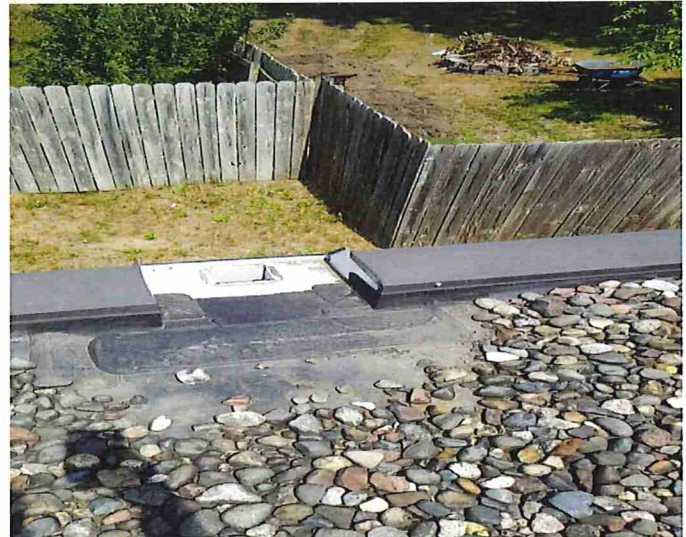
Scuppers are clear of debris.
