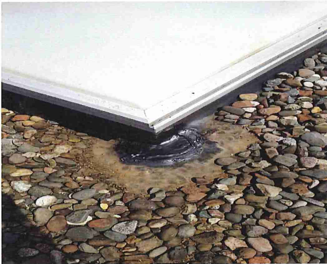
Repaired corner patch.
