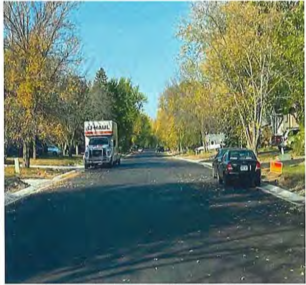
225 th Lane Looking East After Base Course
