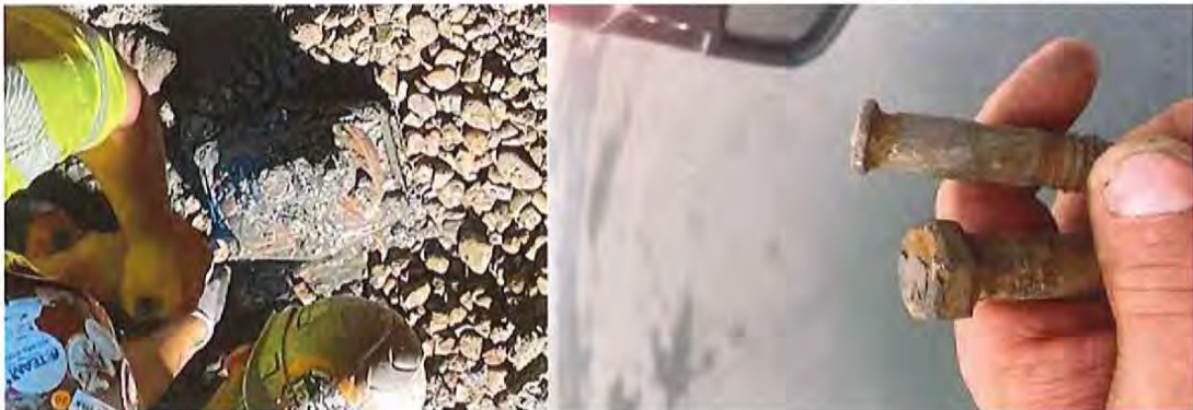
Rum River Blvd- Gate Valve Repair in June.
