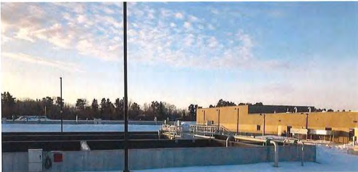
Operation Building and Aeration Tanks
