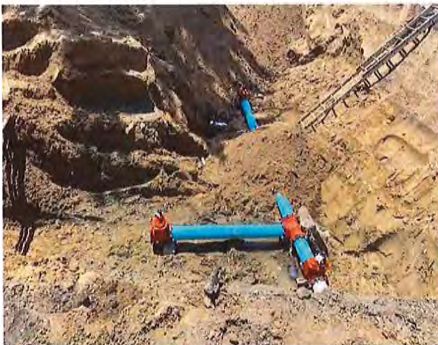
New 8-inch Water Main and Gate Valves
