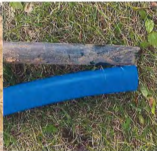
New Water Wervice Pipe, vs Old Pipe
