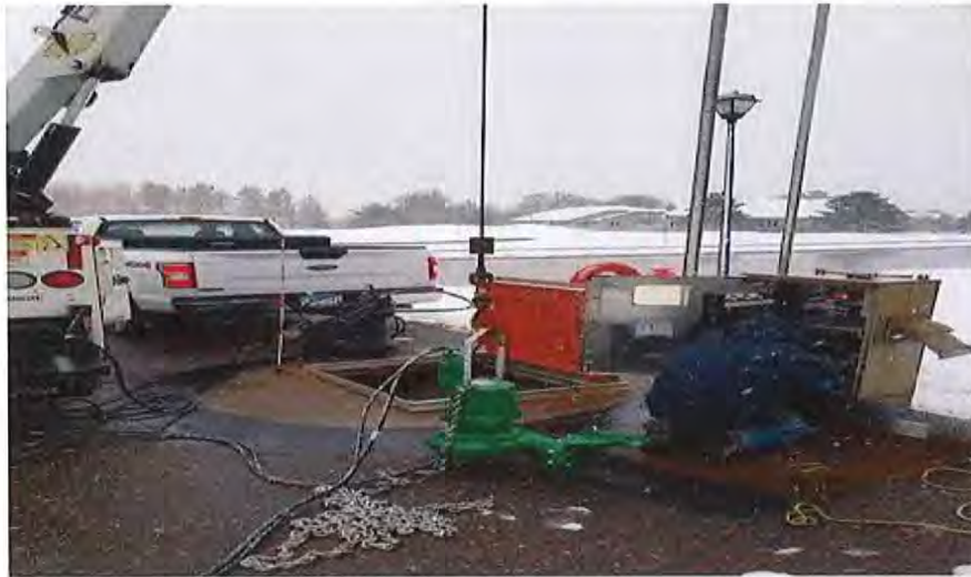
Turtle Run Lift Station-New Pump Install
