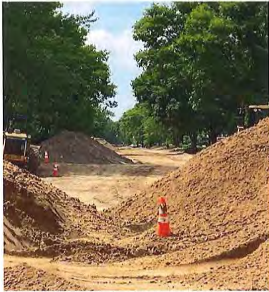
225 th Lane Looking East During Construction
