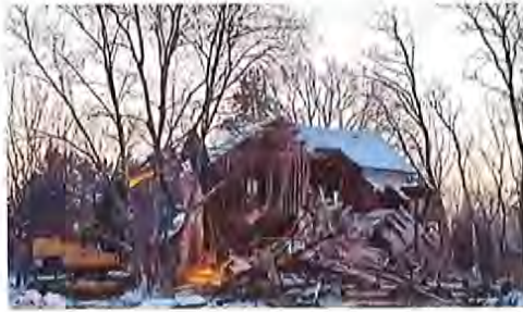
22xxx Rum River Blvd, nuisance property –property was demolished on January 5, 2021.
