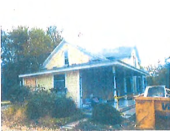
PHOTO #3 Rear Elevation
