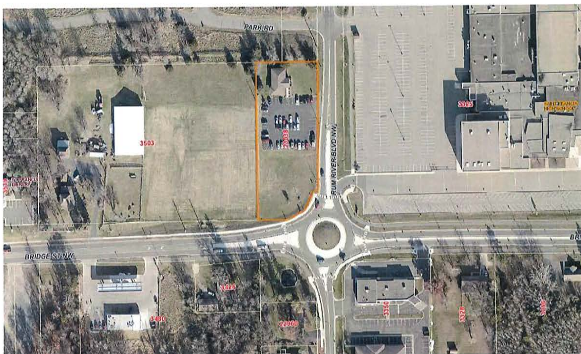
23038 Rum River Blvd is highlighted in orange.
